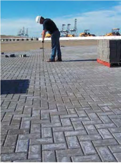
*Straightening of pavers creates straight joint lines and consistent joint widths prior to compaction.*
