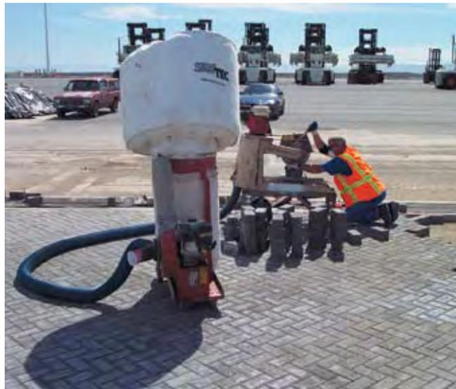
*Cutting pavers to fit at the drains used units no smaller than one third of a paver.*
