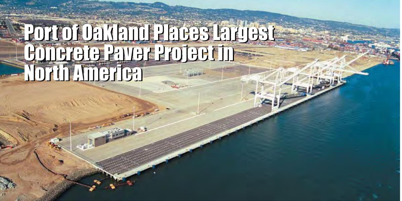
*Berths 55/56 at the Port of Oakland utilizes a record breaking 39 acres (16 ha) of interlocking concrete pavement for container yards. The earth works in the right background (behind cranes) will see an additional 46 acres (19 ha) next year, soon to be another record breaker.*
