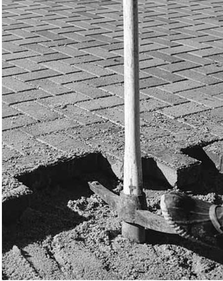
Figure 6. Prying out the remaining pavers
