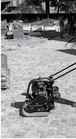
Figure 9. Compacting the pavers and bedding sand.
