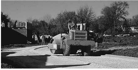
Figure 4. Base compaction with a vibratory roller.
