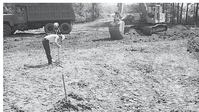
Figure 1. Excavation of the soil subgrade.
