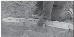
Create a leveling pad of compacted base material that extends a minimum of 6 inches in front of and 6 inches behind the Torpedo base units, that is at least 6 inches deep after compaction.
