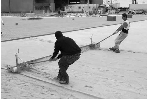
Figure 4. A two-man hand pulled screed
