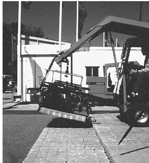
Figure 22. After the layers are separated they can be grabbed by the machine clamp.
