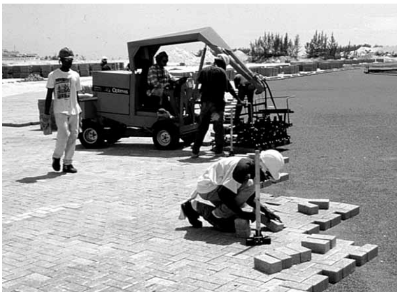
Figure 11. Removal of half pavers and installation of whole units.
