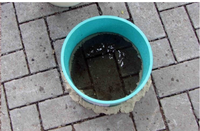
Figure 3. Initial or pre-wetting test using ASTM C1781 permeable interlocking concrete pavement alley. Standing water indicates a clogged surface.
