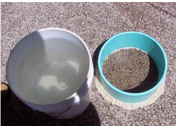
Figure 2. Initial or pre-wetting test using ASTM C1701 on pervious concrete parking lane. Note the standing water due to a clogged surface.
