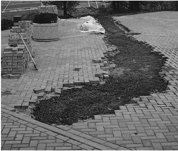
Figure 11. Trench filled with compacted aggregate base. Temporary edge restraints should be used around the opening perimeter.
