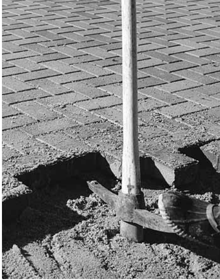
Figure 6. Prying out the remaining pavers
