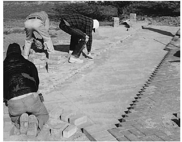
Figure 12. Screeded bedding sand. Note that a few courses of pavers are removed to create even sides for screeding. Installing temporary edge restraints prior to excavating is preferred practice.
