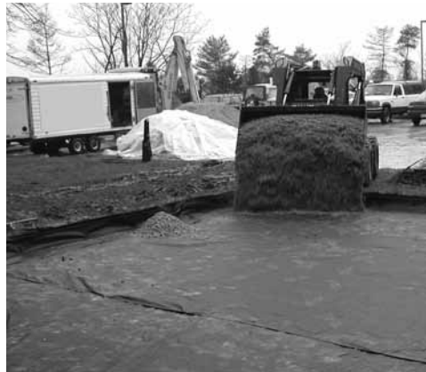
Figure 3. Application of the geotextile under aggregate base.
