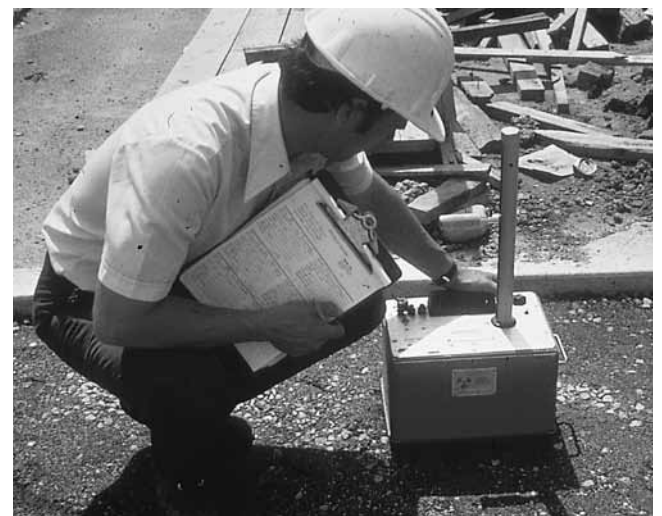
Figure 5. Density testing of the aggregate base with a nuclear density gauge.
