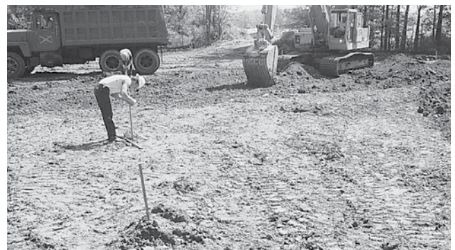
Figure 1. Excavation of the soil subgrade.
