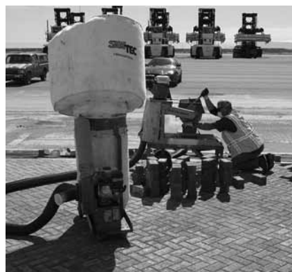
Figure 8. Saw cutting pavers.
