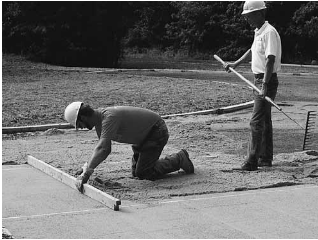
Figure 6. Screeding the bedding sand.
