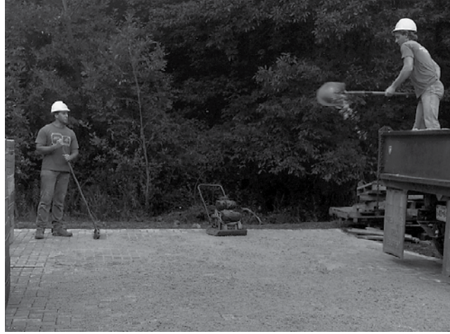
Figure 10. Spreading and sweeping joint sand.
