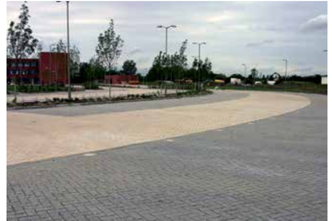
Figures 2 – 5. An example of integrated water and energy design that could emerge from the Integrative Process credit: A horizontal ground source heat pump system is built within a permeable interlocking concrete pavement parking lot. The water in the pavement supports heating and cooling of an office building in the United Kingdom. (Source: Formpave UK)
