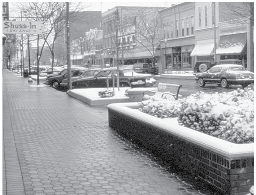
Figure 1. A snow melting system under concrete pavers in downtown Holland, Michigan has performed well since 1988.
