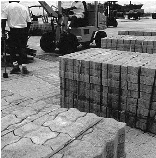
Figure 15. Spacing of cubes at the laying face is determined by how much area will be covered by each, as well as by the clearance required by the machine clamp. Orientation of the cubes follows the direction of paving.
