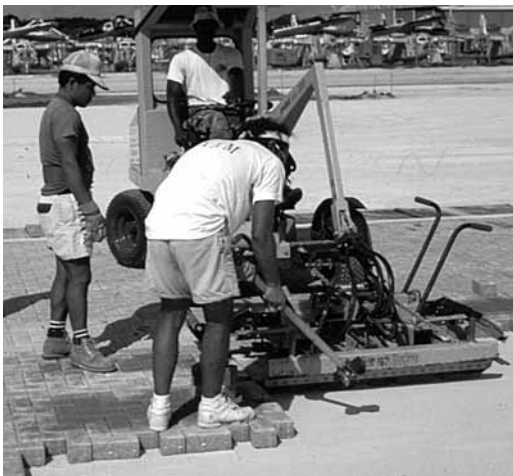
Figure 5. Motorized equipment with a hydraulic clamp.
