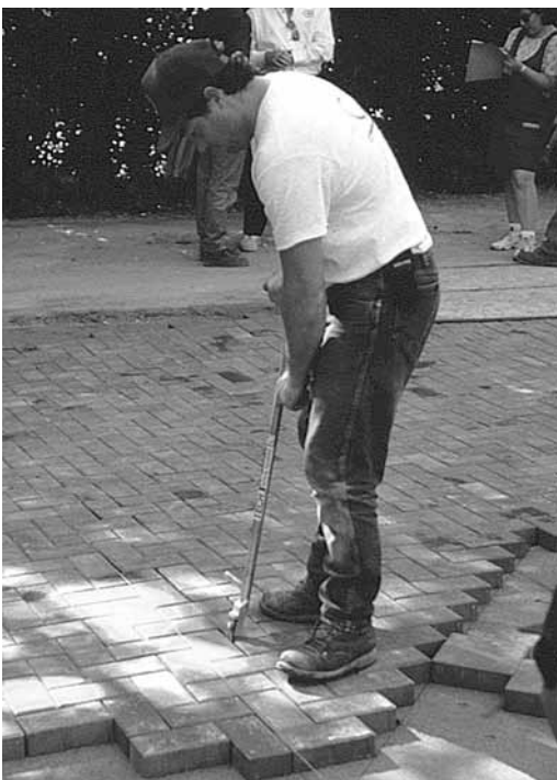
Figure 20. Adjusting joint lines with a pry bar prior to compaction.
