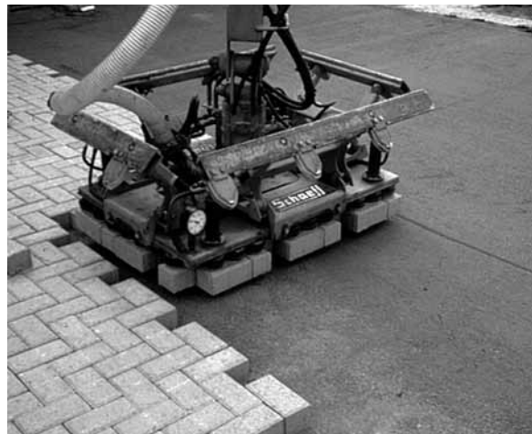
Figure 6. The vacuum head over the paver layer.
