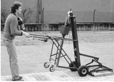
Figure 3. Non-motorized equipment used to set a small layer of pavers.
