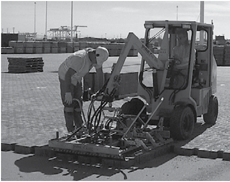
Figure 9. Mechanical installation equipment places concrete pavers rapidly.
