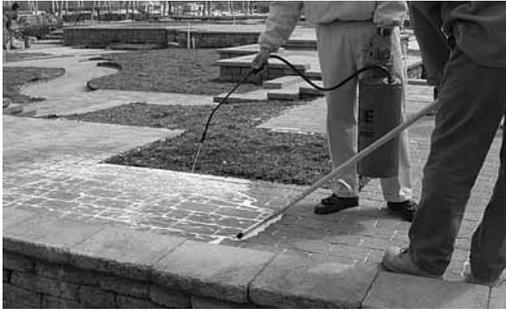
Figure 3. This liquid joint sand stabilizer is applied with a low-pressure sprayer and squeegeed across the surface after allowing some time for soaking into the joints. This helps maintain slip and skid resistance of the paver surface.
