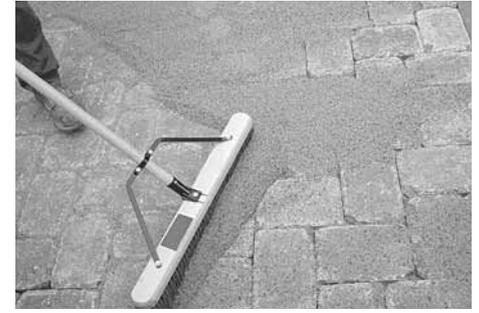
Figure 5. Joint sand can be pre-mixed and delivered to the site (typically in bags), or mixed with stabilizer at the site, then swept into the joints, compacted for consolidation in them to create interlock, and wetted to activate the stabilizer.
