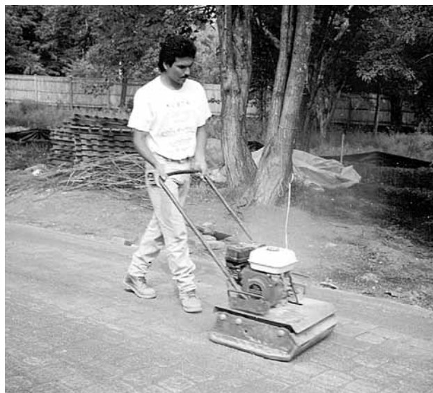
Figure 9. Final compaction of the pavers and settling of the sand into the joints.
