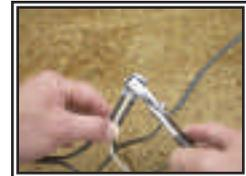
10. Repeat steps 8 & 9 using the smooth sides of the power supply cable and the white wire from the light. You should end up with two connections per light as shown. **After all lights have been attached, plug in and switch on the transformer to test all connections.**
