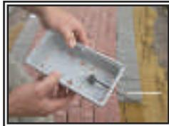
6. Run the low voltage cable which will supply power to the lights around the perimeter of your project. For installation with segmental pavers, you may set the cable atop the bedding sand under the border course of pavers to keep it from being damaged when digging in the yard and so it can be easily located. Form a loop in the cable where the lights will be located (with a rubber band if desired) to leave enough slack for connection of the light to the power cable.
